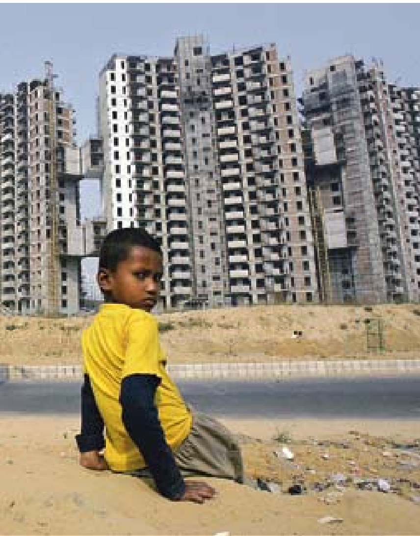
Idle cranes . . . construction sites the world over – this one is in Gurgaon, India – have been halted by the financial crisis Gurinder Osan/AP
